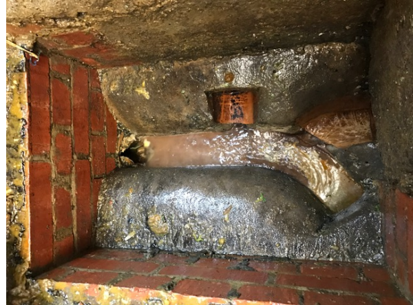
Manhole after emptying
