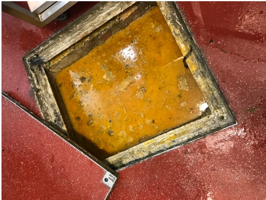
ManholeX_b21ca32d-01aa-47bb-a639-343f595d82d9_20170404_174927.jpg, 00:00:00, 0.00m Start node type, manhole, reference number: Manhole
