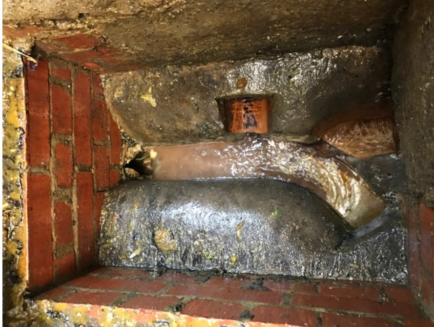
ManholeX_5b8418f4-9878-4034-bf0f-26c0b27ca98c_20170404_175008.jpg, 00:00:00, 0.00m Start node type, manhole, reference number: Manhole
